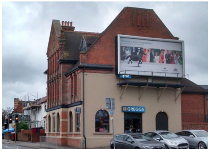
Illuminated advertising on the upper northern elevation of the former Wellington Arms
