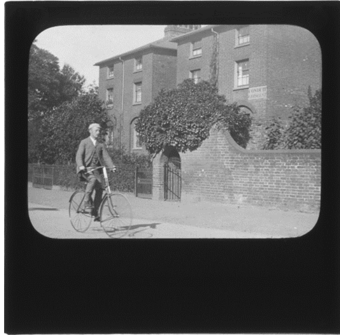
Conduit Crescent C 1910. Lantern slide from Reading Museum. Mr Cox on his bicycle. Note archway through to conduit. Museum object number REDMG: 1931.435.62
